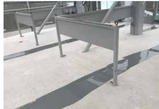
CRACK TREATMENT
