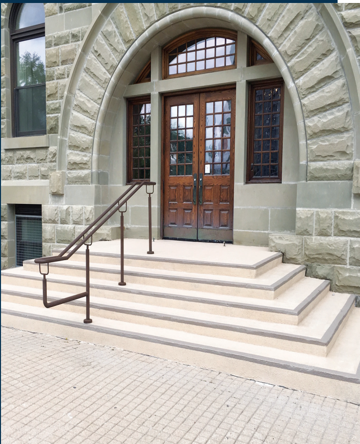
EXTERIOR STAIRS Stonwalk
