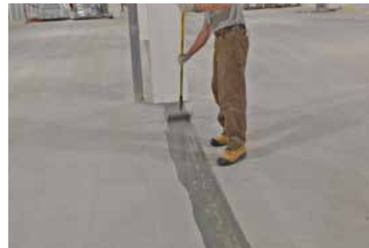
CRACK TREATMENT
