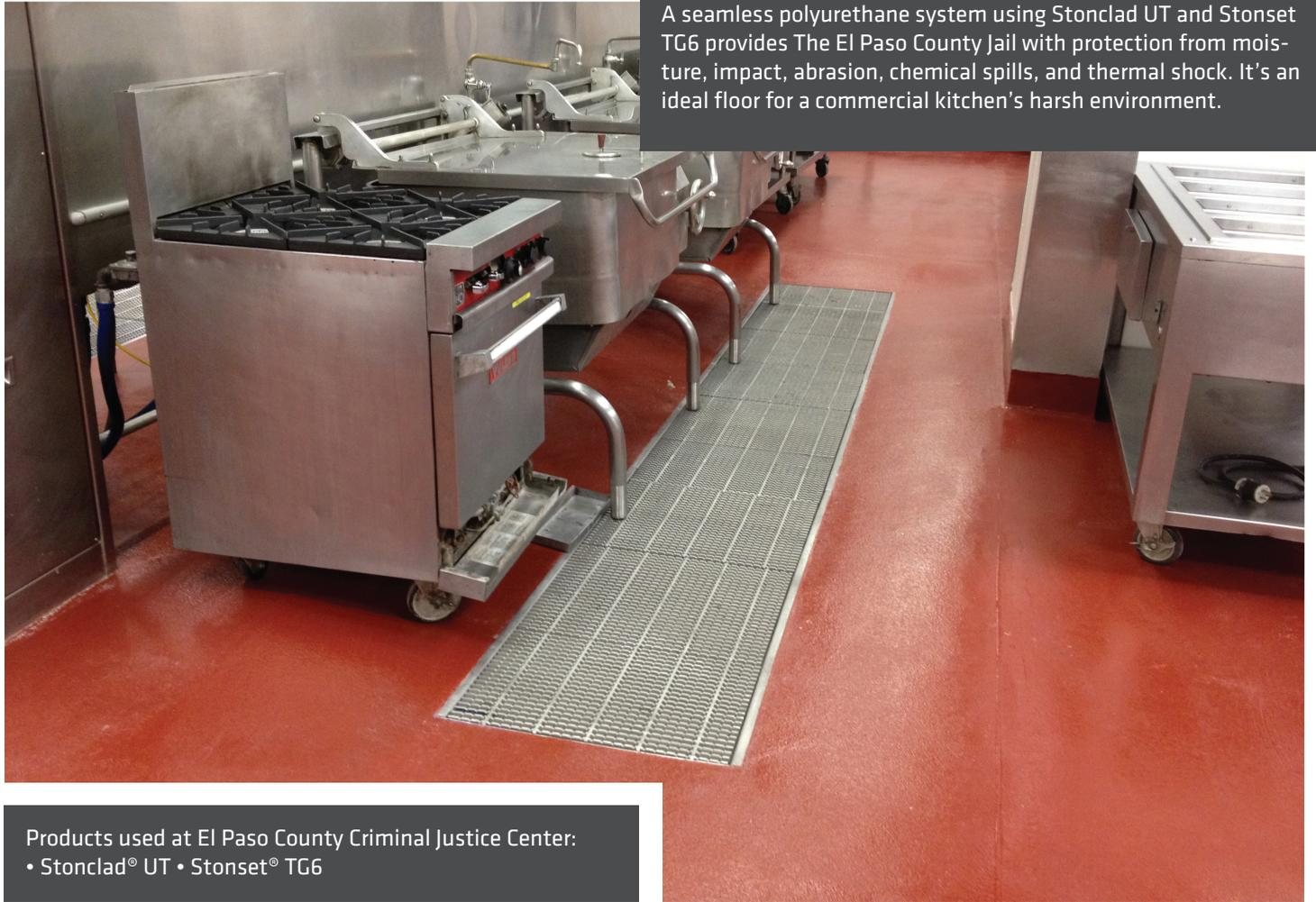
A seamless polyurethane system using Stonclad UT and Stonset TG6 provides The El Paso County Jail with protection from moisture, impact, abrasion, chemical spills, and thermal shock. It's an ideal floor for a commercial kitchen's harsh environment.
