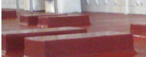
Stonhard's Stonblend GSI-G system incorporates recycled glass into its composition and provides a durable, easy-to-clean, decorative floor for offices, labs, locker rooms and break rooms at Shearer's.
