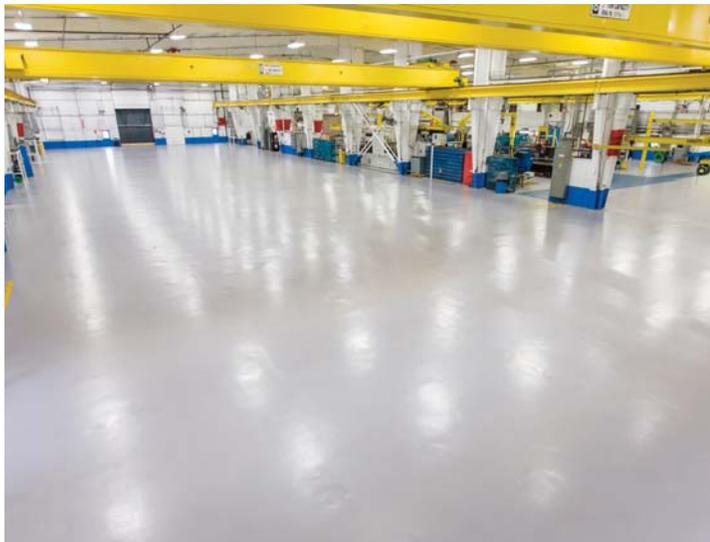
*Stonclad GS replaced severely worn, oil-soaked concrete*
