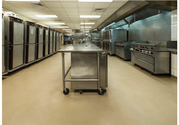
The worn quarry tile in the kitchen and concession areas were replaced with seamless, easy to clean, stain resistant Stonclad
